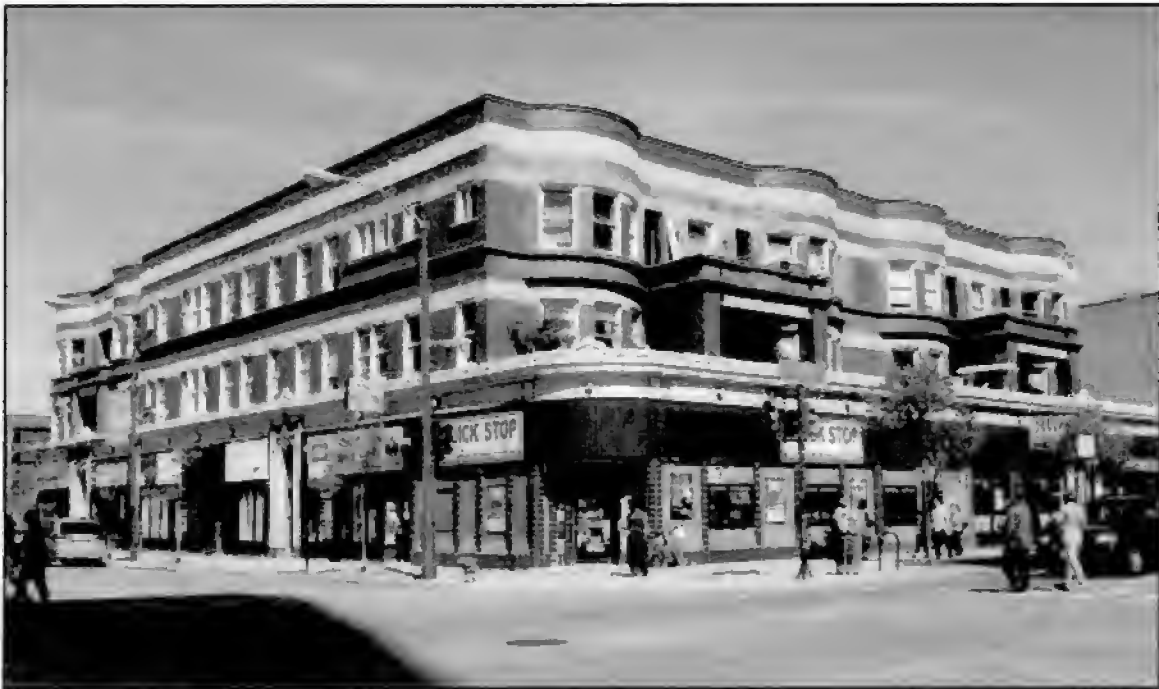
1000-1010 West Argyle Street (1908 with c. 1915 with later storefronts)
